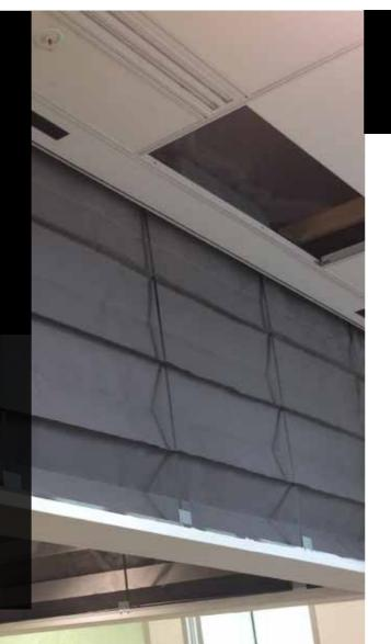
The unique features of the SmokeStop Concertina allow it to be used in place of traditional smoke control elements, allowing architects, fire engineers and specifiers to create open plan designs which meet all the requirements of a building's smoke control strategy.
