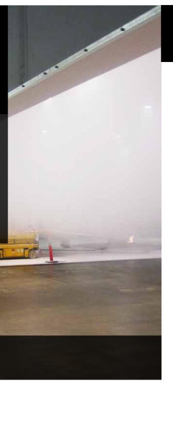
SmokeStop Smoke Barriers are designed as barriers to prevent the spread of smoke in accordance with BS EN 12101-01:2005+A1:2006 and are classified as either DH60 or  $\mathsf{D}_{_{600}}\mathsf{A}.$  SmokeStop is legally CE Marked in accordance with the Construction Products Regulations.
