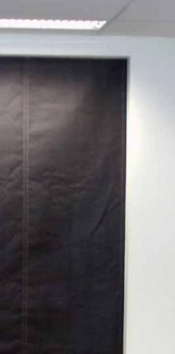
The Vii Fire iZone product is designed as a barrier to prevent the spread of fire in accordance with BS EN 1634-1:2008 and BS 8524-1:2013 for such applications as protecting Means of Escape and achieves E180 EW60 (180 mins integrity and 60mins radiation).
