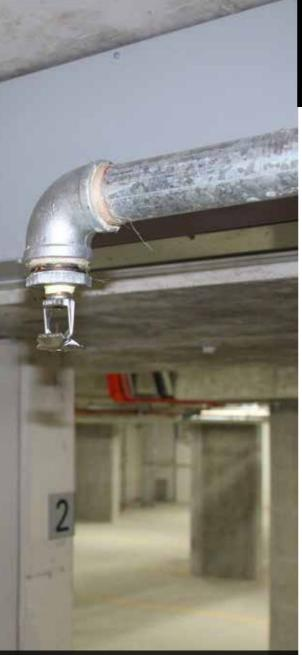
Positioning, alignment and selection of the correct sprinkler heads is critical with only simple connection to a suitable water supply. FireMaster SuperPlus is designed to prevent the spread of fire in accordance with BS EN 1634-1:2008.
