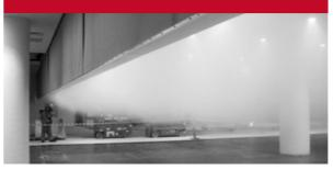
Coopers Fire full range of fire and smoke curtains can be used to create compartments to contain fire and smoke and prevent it from spreading. The product range is used particularly in this instance in large open spaces in buildings.
